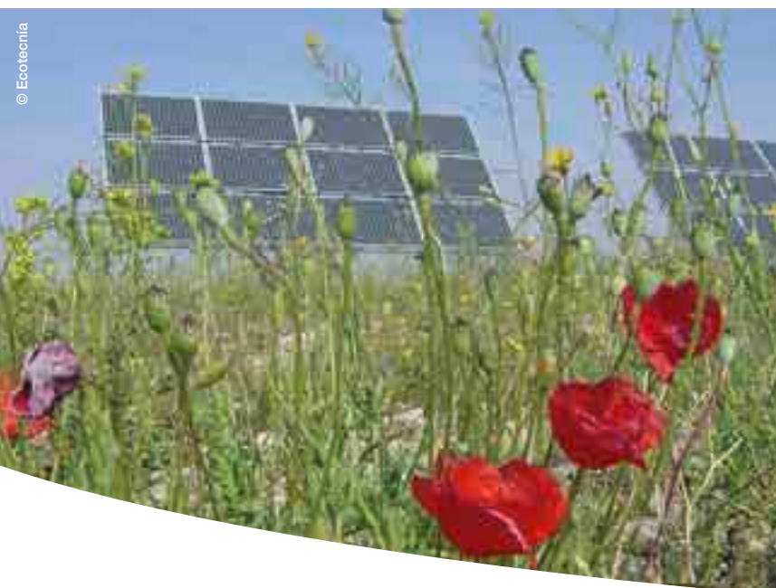
Large solar power plant in Spain
