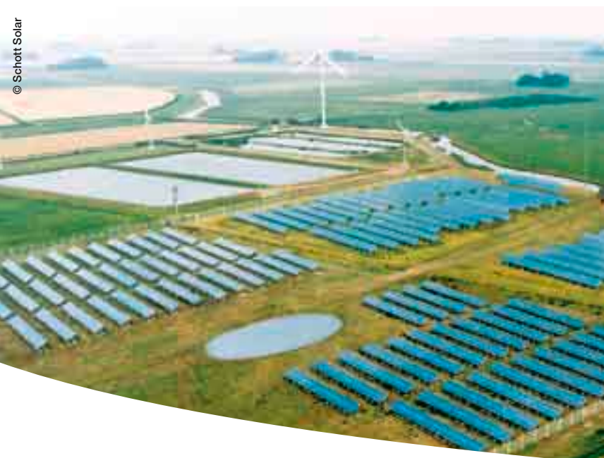
PV plant in Pellworm
