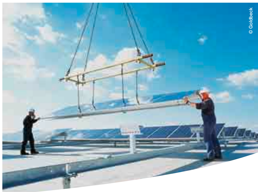
Installation of modules on a building roof
