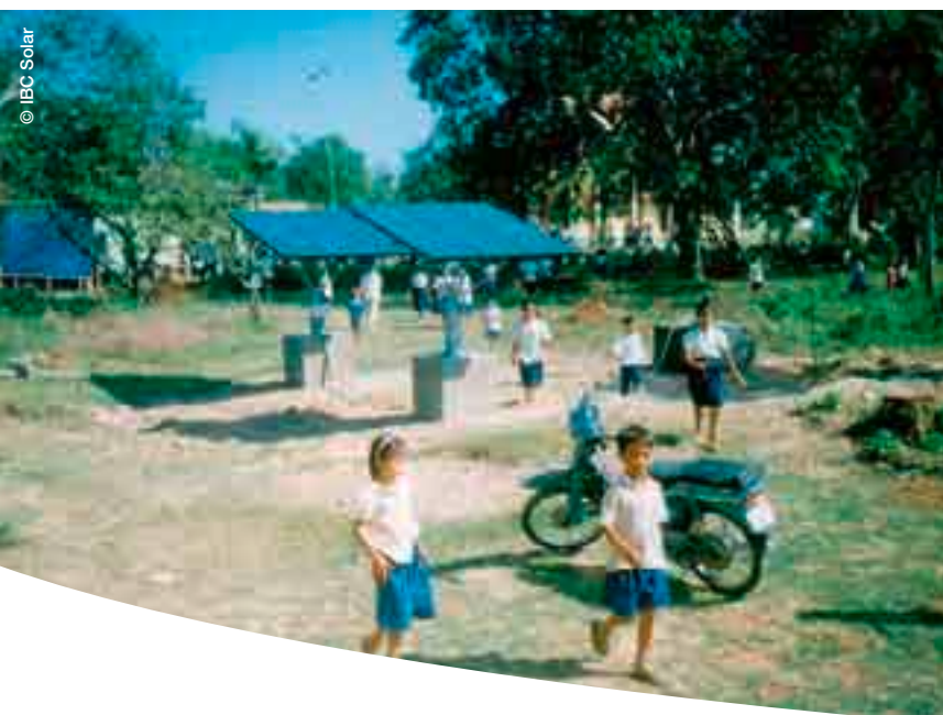
PV system in a school in Cambodia
