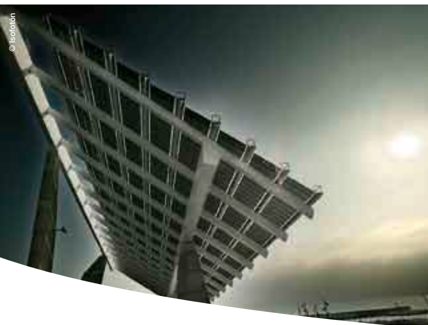
PV pergola on the Forum in Barcelona
